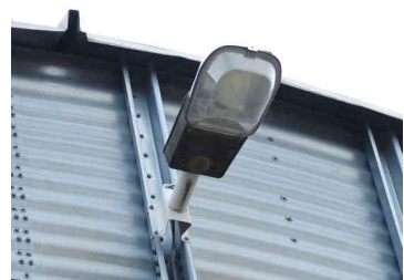
Figure E.15: NonFCO, clear glass. UH: 0%, UL: 5- 10%, ULR: 5-10%
