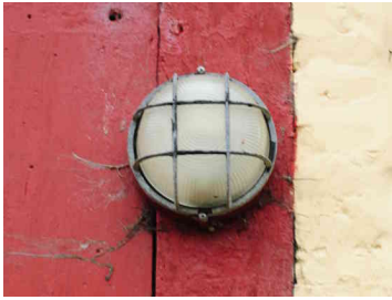
Figure E.17: NonFCO, frosted plastic, UH: 41% UL: 9%, ULR: 50%
