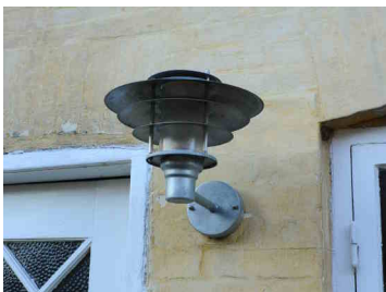
Figure E.33: NonFCO, frosted glass, UH: 0% UL: <5%, ULR: <5%
