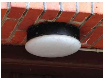
Figure E.10: NonFCO, frosted glass. As installed in this figure, UH: 10-15%, UL:5-10%, ULR: 15%-25%. This type of fixture is often installed vertical on walls, then the ULR increases to 50% with UH: 41%, UL: 9%.
