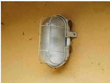
Figure E.20: NonFCO, frosted plastic, UH: 41% UL: 9%, ULR: 50%
