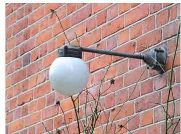
Figure E.14: NonFCO, frosted glass. UH: 33 - 35%, UL: 8 -10%, ULR: 42 - 45%
