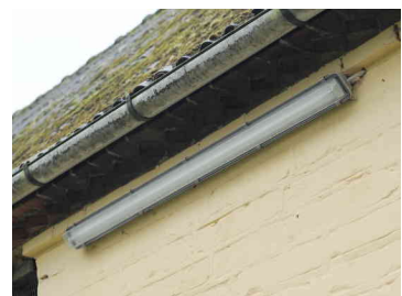
Figure E.16: In the figure the fixture is angled approx- imately 45° from horizontal. It is possible to find this kind of fixture installed in any angle from horizontal (0°) to 90°. Due to the different angles of installation the fixtures ULR varies considerably. UH: <10 - 41%, UL: 5 - 9%, ULR: <15 - 50%.
