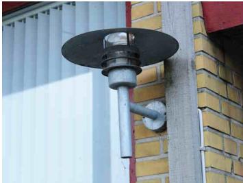
Figure E.31: NonFCO, clear glass, UH: 15 - 35% depending on the installed light source. UL: 5 - 10% ULR: 20 - 45%
