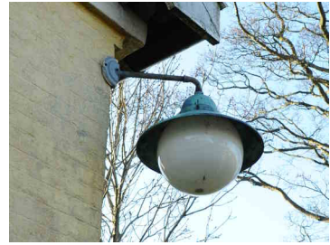
Figure E.35: Rare historic fixture, nonFCO, frosted glass, UH: 5% UL: 9%, ULR: 14%
