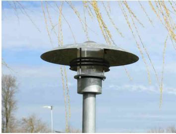
Figure E.6: NonFCO, clear glass, UH: 15 - 35% depending on the installed light source. UL: 5 - 10% ULR: 20 - 45%
