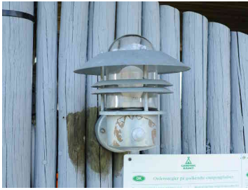
Figure E.5: NonFCO, clear glass, UH: 15 - 35% depending on the installed light source. UL: 5 - 10% ULR: 20 - 45%
