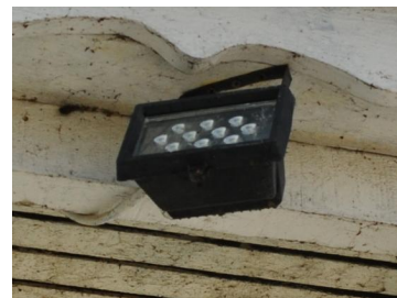
Figure E.1: NonFCO, LED projector. Fixture is not FCO and the CCT is to high >3000K.
