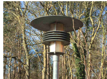
Figure F.2: NonFCO, clear glass, UH: <5% UL: 9% ULR: 10-14%.
